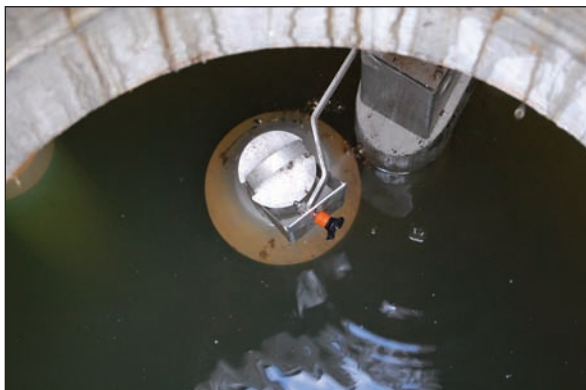
ecoStop ® valve and float in "open" position
